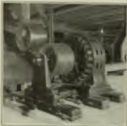
FIG. 1. MOTOR DRIVEN, AN 8-FOOT MILL, 130 HORSEPOWER
